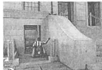
A new elevator entrance was provided next to the stairs to provide universal access to the services inside. Photo: Courtesy, GSA.
