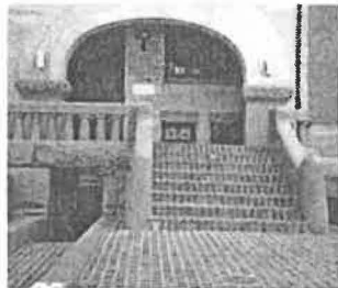
A significant entrance may be difficult to modify. Although a special challenge, sensitive changes can almost always be made to provide access while preserving the unique historic character. Photo: NPS files.
