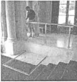
A retractable lift for this historic building foyer was created using "like" materials. Photo: NPS files.
