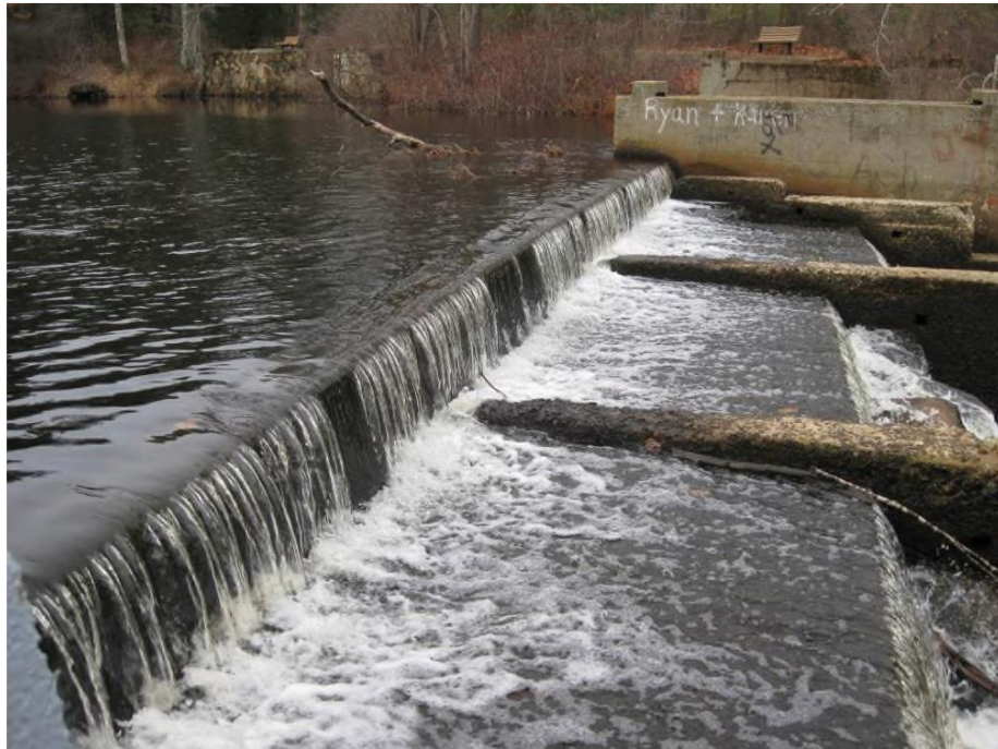
Figure 12: Curtiss Crossing Dam, primary spillway weir (right)
