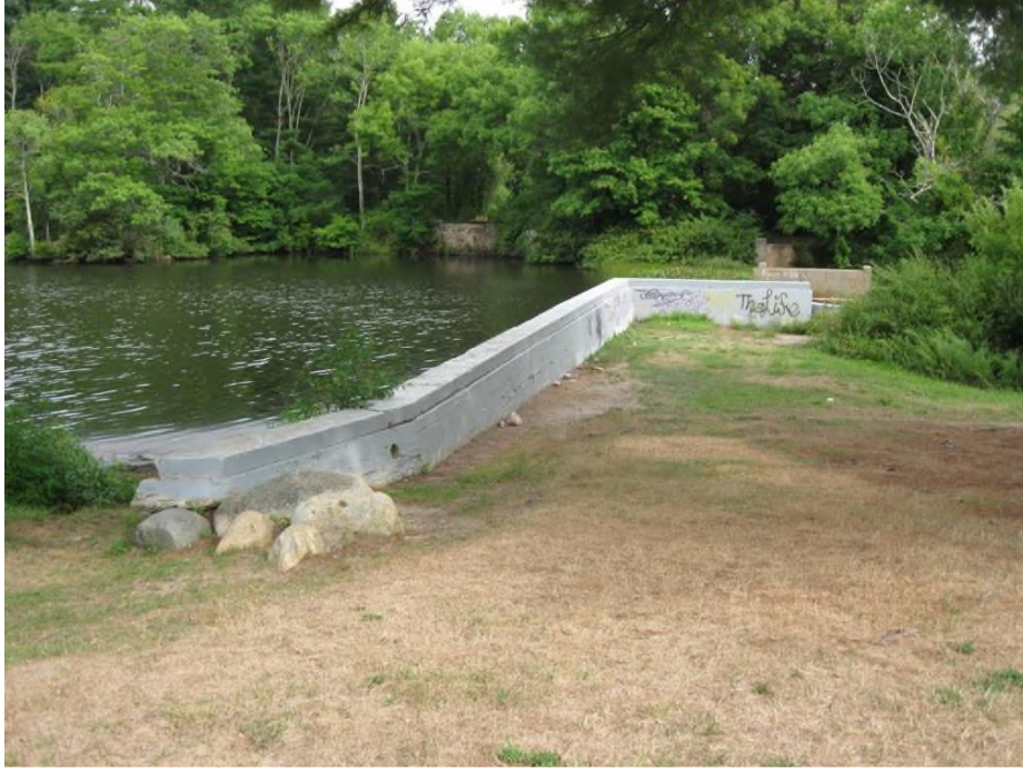
Figure 11: Curtiss Crossing Dam, Crest from right abutment
