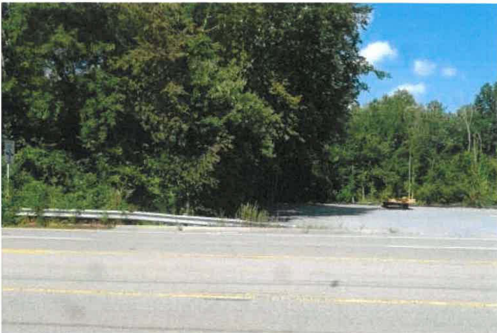
Right Side of Subject Property – Looking Northerly Photographs Taken by M. Tyburski on September 6, 2021
